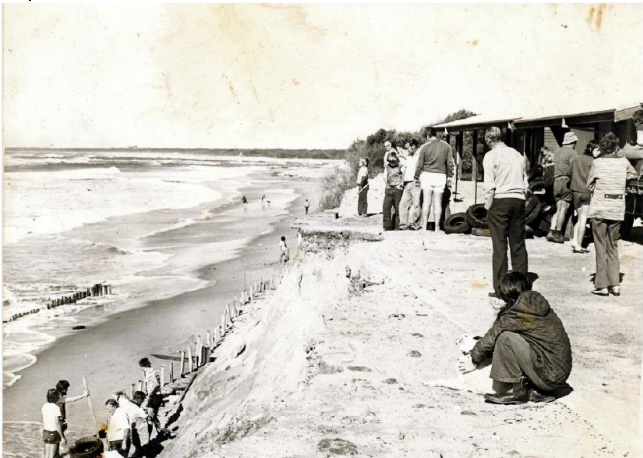
Figure 10. Shoalhaven Heads Surf Club construction of rock revetment, circa 1978 (source: BMT WBM 2012)
